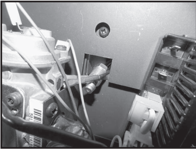
Figure 68: Square slot for insertion and removal of pilot assy.
