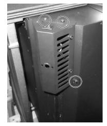
2 Tilt the assembly down being careful not to damage the wires connecting the assembly to the unit. Unscrew the (2) screws on the side of the assembly to remove the heatshield and expose the wiring. Set the screws aside for reinstallation.
