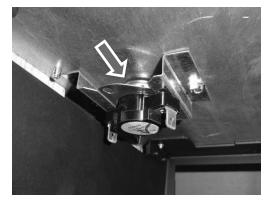
7 Place the blower assembly on the floor behind the stove close enough that the wires on the assembly can reach the snap disk on the stove. Locate the two black wires on the blower assembly labeled "Snap Disk" and connect them to the terminals on the snap disk (polarity does not matter).
