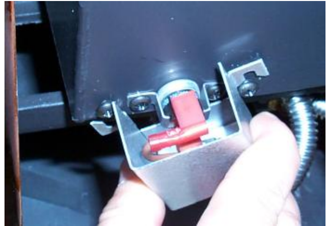
Photo #6 – Snap Switch Protective Cover Installation
