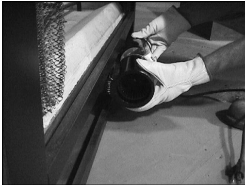
Figure 4 - Inserting the Fan into the Fireplace
